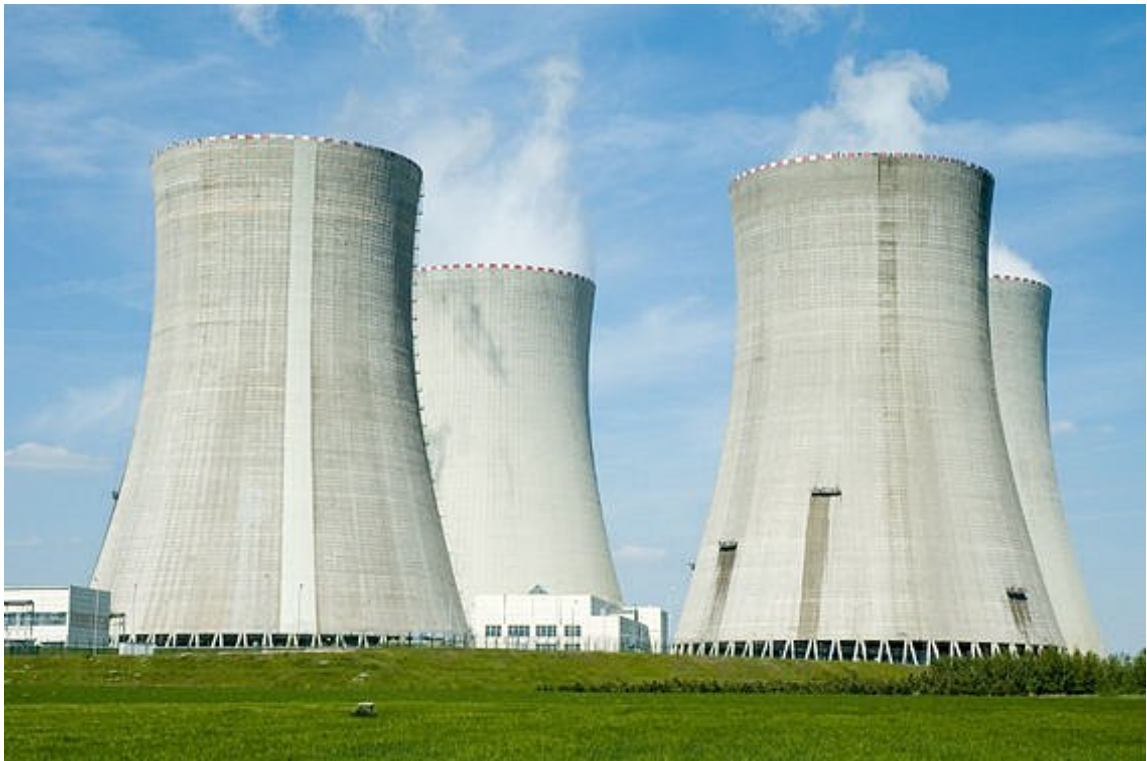
Figure 1: Typical cooling tower
